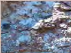
Brockram (seen here in a wall in Kirkby Stephen) is made of fragments of Carboniferous limestone set in red siltstone and sandstone. It formed in alluvial fans in Permian desert landscapes.
