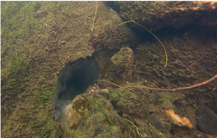
One of the underwater voids showing water being sucked in.
