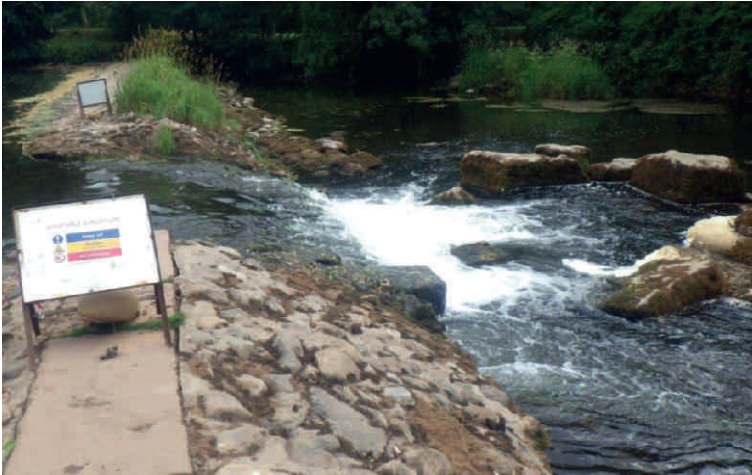
Above/bottom left: Middle of the weir washed away and broken pieces of the fish pass scattered downstream. Photo: O Southgate
